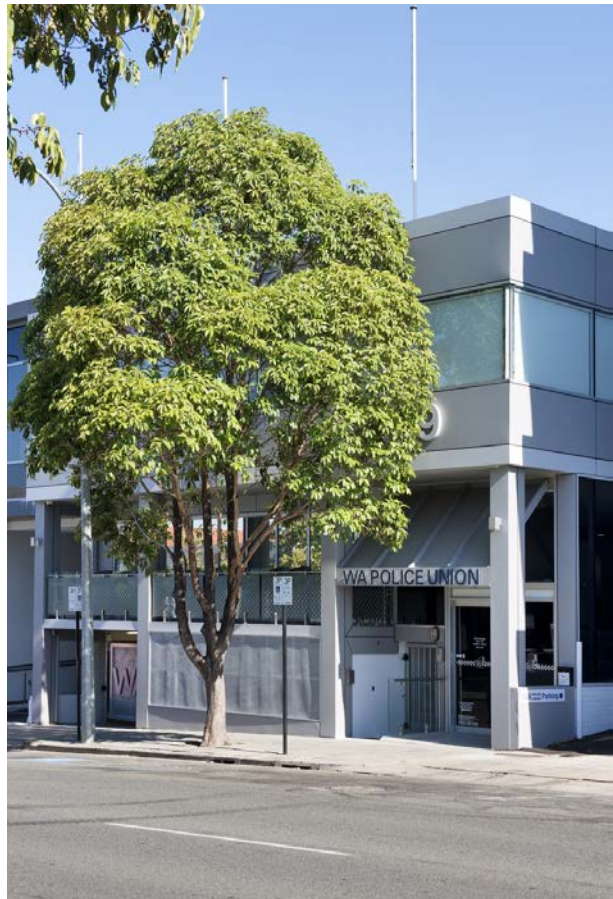
External view of the refurbished WAPU HQ on Murray Street
